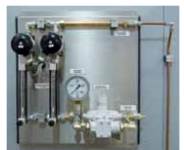
Gas supply system for HFL 160/17
