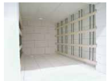
Protective screen in front of heating elements for protection against mechanical damage
